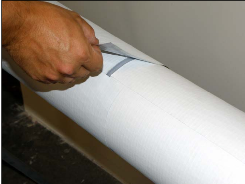
Photo 1: Butt strips applied to circumferential joints
